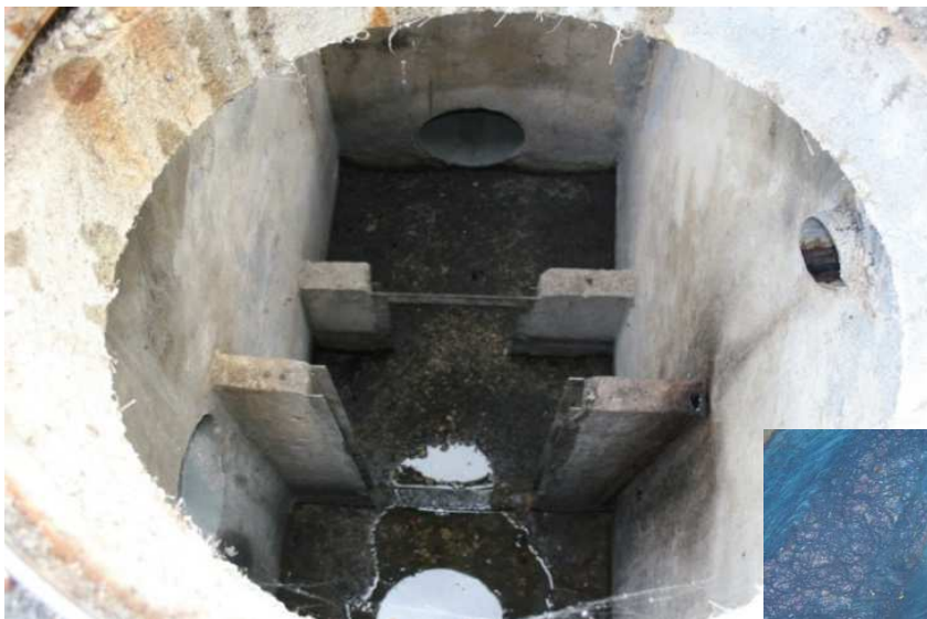
Inflow sabotaged (missing valve) © Bourgogne, 2010
