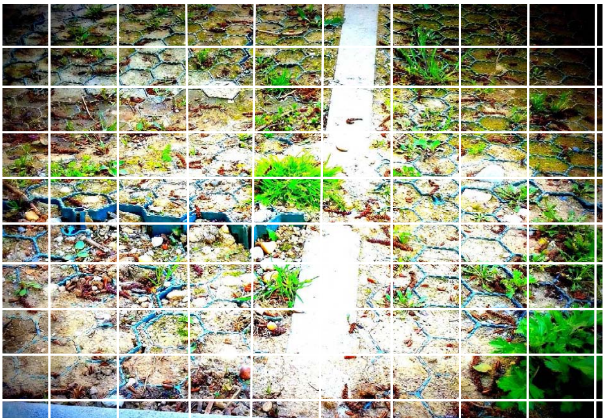
Parking perméable endommagé © Cherqui, 2015
